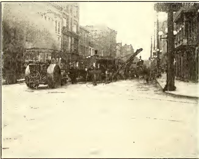
ELMIRA TRACK RECONSTRUCTION—FIG. 8—STEAM SHOVEL AND STEAM ROLLER AT WORK; STRETCH OF FINISHED TRACK IN FOREGROUND
